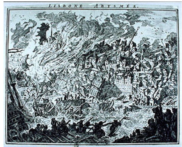
Figure 3. The Great Lisbon Earthquake
